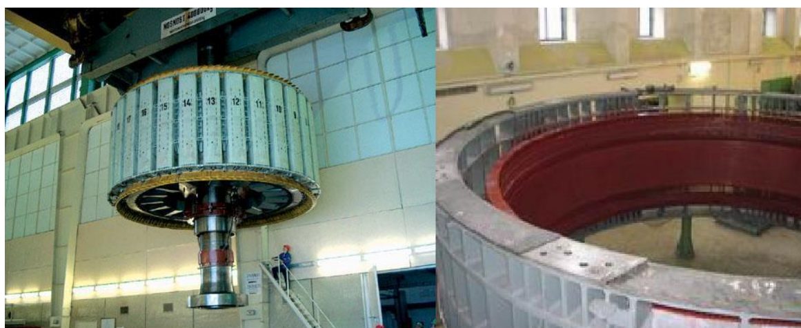
Fig. 6.2 Stator and rotor of hydroalternator (Štěchovice power station)
