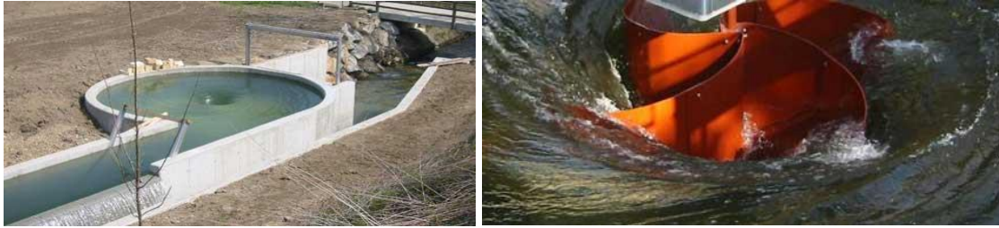
Fig. 4.14 Left: vortex power plant, Right: Zotlöterer turbine
